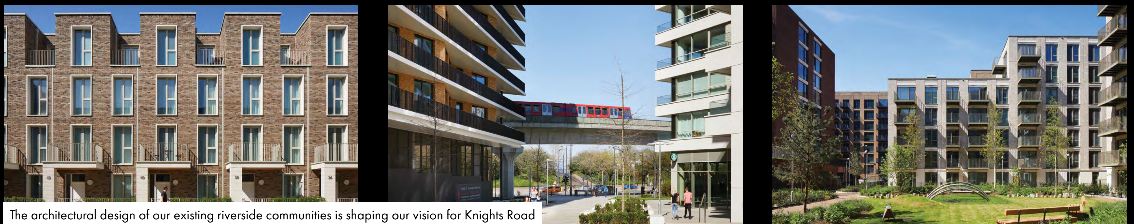
The architectural design of our existing riverside communities is shaping our vision for Knights Road
